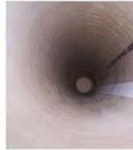
Cured in Place Pipe provides a new liner that stops root infestation and provided additional structure to the pipe.
